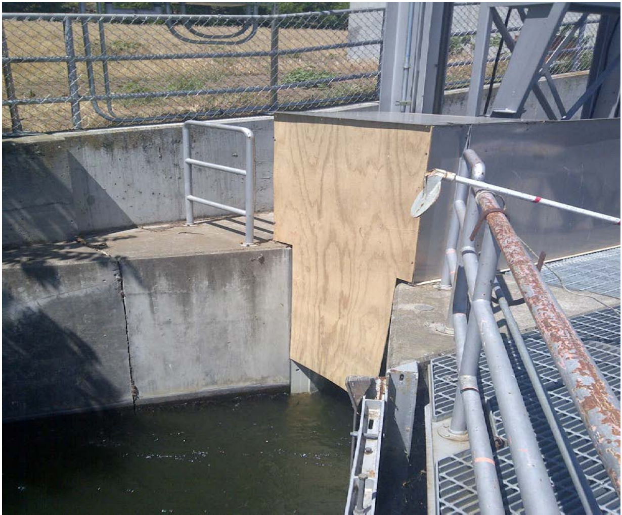
Wood panel sunshade installed at north count station to replace aluminum in attempts to reduce PIT antenna interference.
